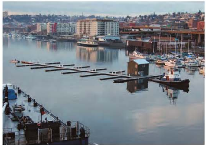
Once Marine Floats completely built the renovated dock, it barged the dock down the river to the marina.
